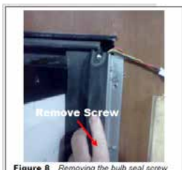
Figure 8 Removing the bulb seal screw
