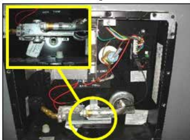
Fig 1: Water Heater Drain Plug
