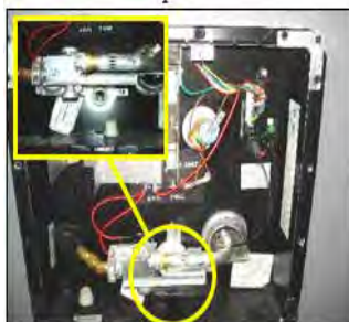
Fig 1: Water Heater Drain Plug
