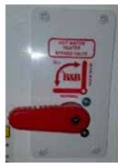
Water Heater Bypass
