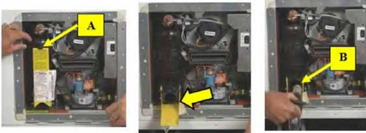
Draining the Aqua Go Water Heater
