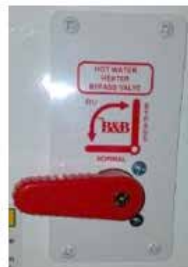
Water Heater Bypass
