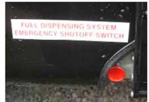
Master/Emergency Fuel Disconnect Switch locations
