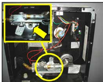
Water Heater Drain Plug Location
