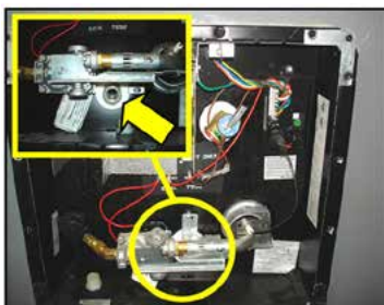
Water Heater Drain Plug Location
