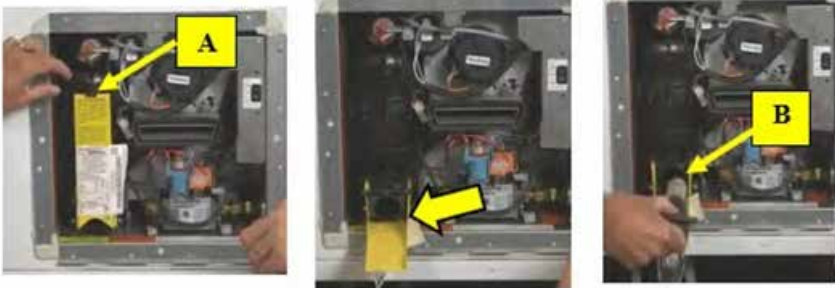
Draining the Aqua Go Water Heater
