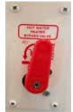
Water Heater Bypass
