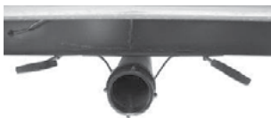
Black/Grey Tank Drain and Valves
