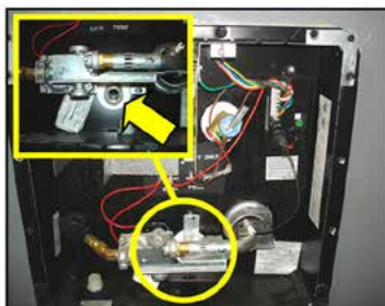
Water Heater Drain Plug Location
