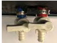
Low Point Drain Example
