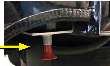
Master/Emergency Fuel Disconnect Location
