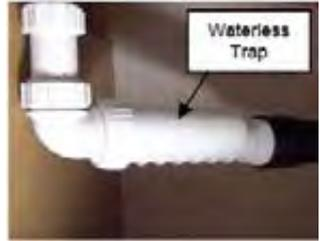
**REMOVE WATERLESS TRAP BEFORE
