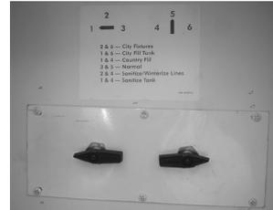
Fig. A -Water Valve Controls
