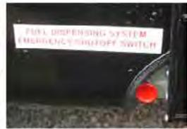
**NOTE:** This switch should be “OFF” position (knob pushed in) when the fuel station is not in use.
