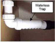
piping to open the drain. Passing a cleanout tool through the waterless valve may cause damage to the internal seal that may potentially allow sewer gases to escape into the RV interior. The waterless trap can be unscrewed from the water lines. A label has been placed near the location of the waste valve that reads as follows:
