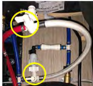
Water heater Bypass Access shown in NORMAL mode
