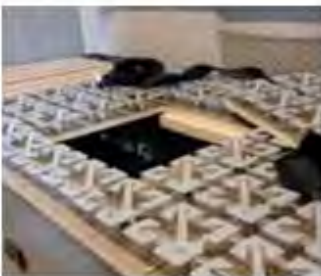
Water heater Bypass Access
