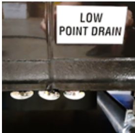
Low Point Drain Example
