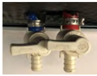
Low Point Drain Example
