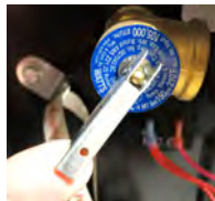
T&P Relief Valve Example
