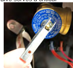
Water Heater Pressure Valve
