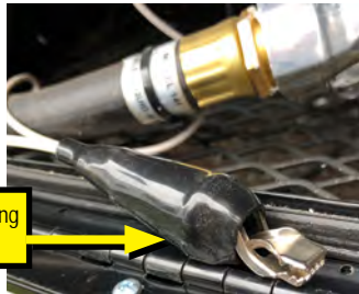
Grounding Clip Inside Fuel Station
