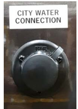
City Water Fill w/Connection Label
