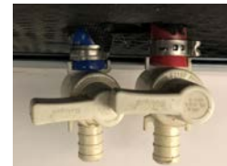
Low Point Drains - Some Models
